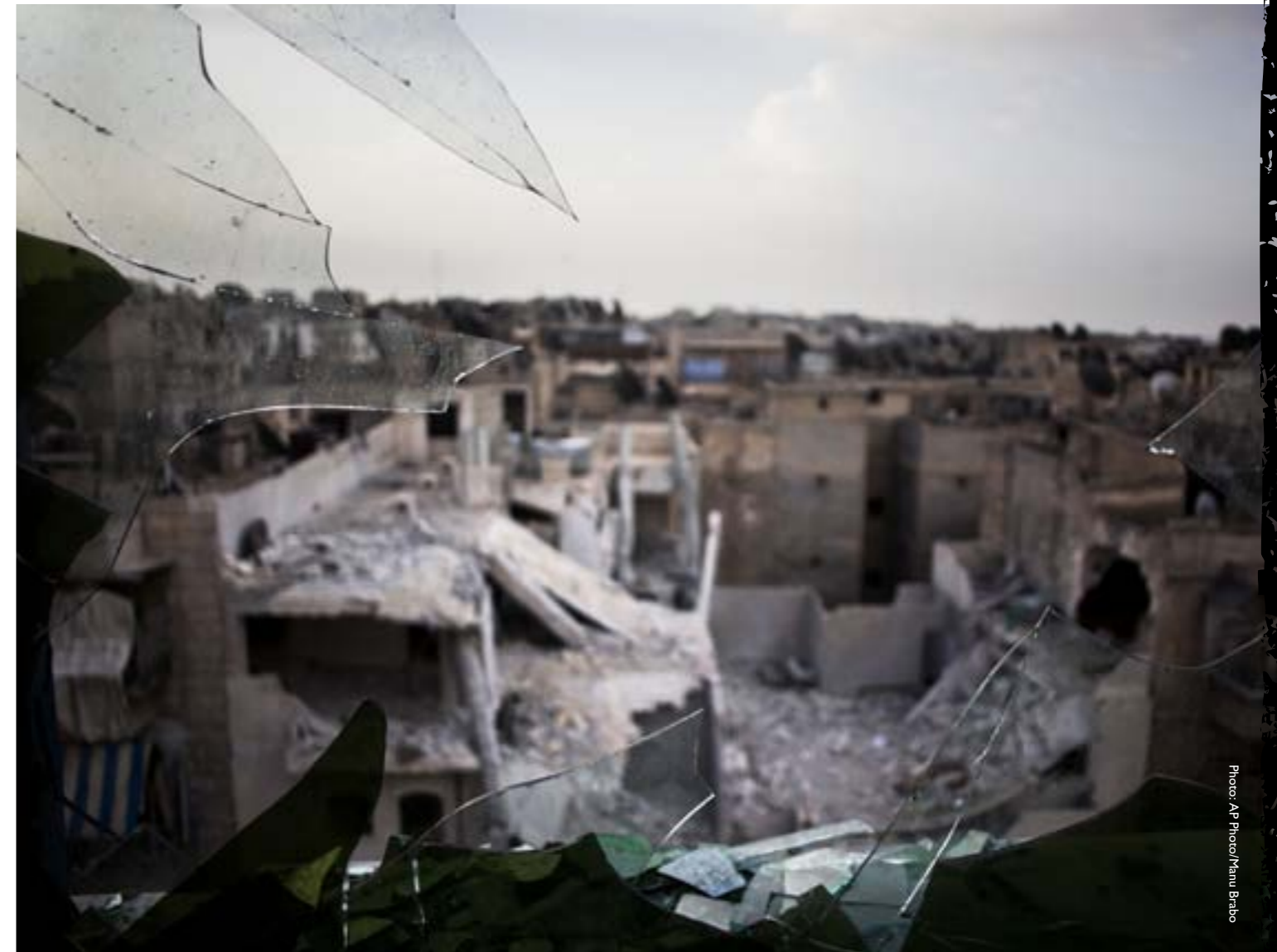
Buildings damaged by shelling in Aleppo, Syria.
